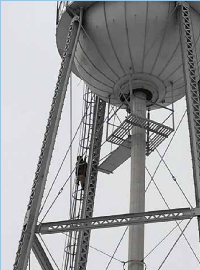
The contractor climbing into Hannaford tank to steam the frozen intake.
