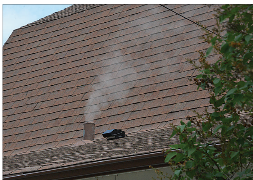
Pictured above, crews hook up the equipment to run the smoke testing. Below, the smoke rises from a house in the way it should if things are properly vented.
