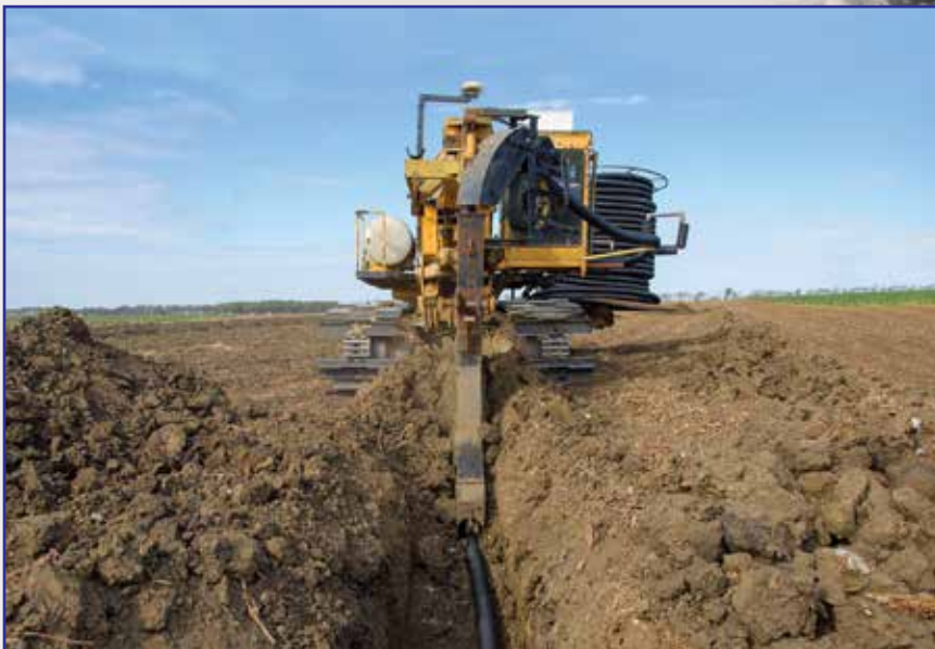
A drain tile being installed into an agricultural field.
